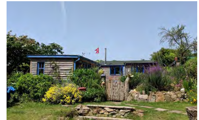
Below: Chalet at Holts Field
