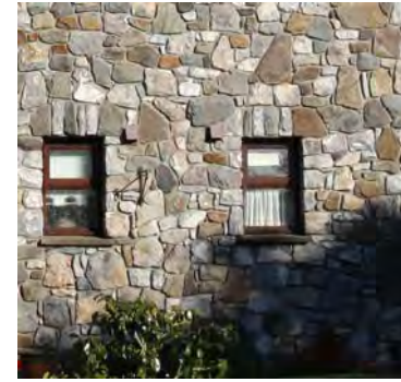
Above: 20th century development which has used stonework to relatively good effect, however more attention to the placement of the stones would have enhanced it further
