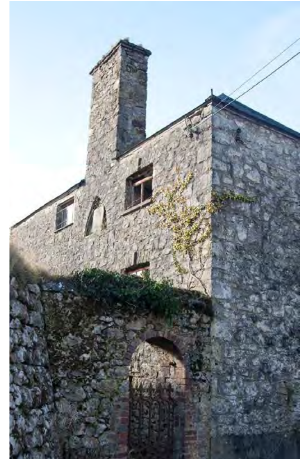
Above: Lower Mill, Llanrhidian: Grade II
