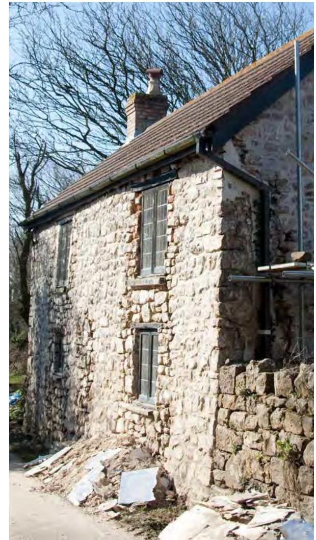
Above: Restoration works in progress, Middleton
