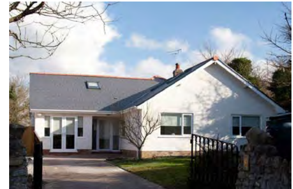
Above: recently renovated adjacent property
