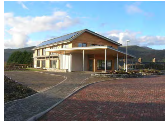
Above: Commercial development, Dyfi Valley, JPW
