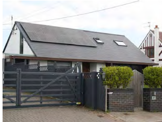
Above: Photovoltaics to roof, Southgate
