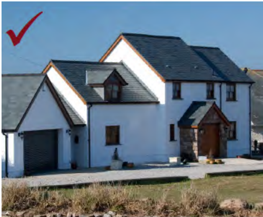
Above: Sub-dividing a house into a number of visually distinct elements can reduce its overall visual impact, creating a more sensitive form of development
