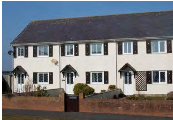
Above: examples of twentieth century suburban style development found in Gower
