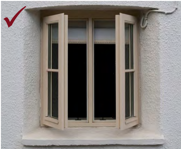
Above: timber opening casement painted window
