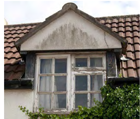
Below: poorly maintained windows can detract from the overall appearance of a building as well as allowing water to penetrate the structure.
