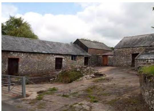
Below: farm buildings used as basis for the preparation of illustrative examples ( right )
