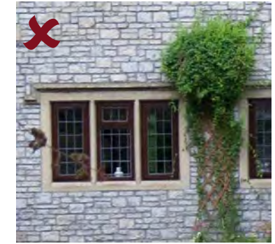
Above: 20th century development which has poorly chosen stone, in terms of both colour and size, and inappropriate mortar colour and pointing style
