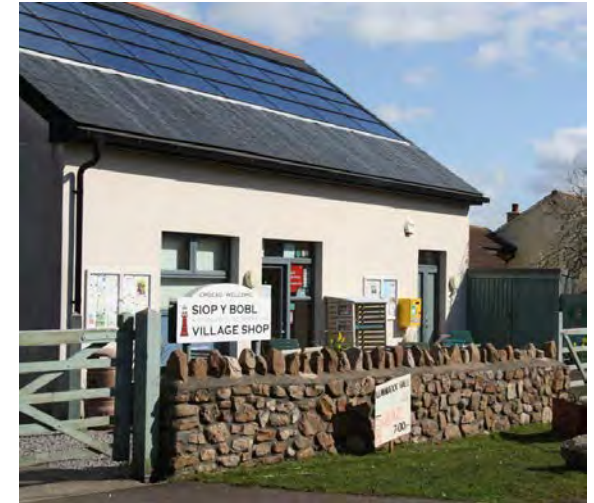
Above: PV installation Llanmadoc
