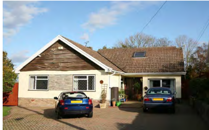
Above: largely original, well maintained 1970's bungalow, with additional rooflight
