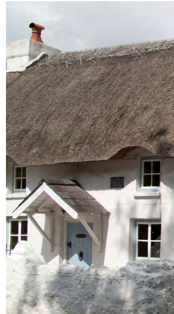
Above: The Nook, Oxwich: Grade II
