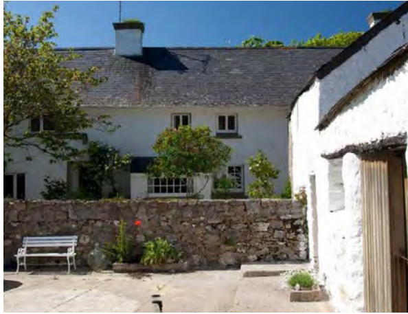
Above: Great Pitton Farm, (Grade II listed), is an example of traditional Gower Farmhouse with small windows and slated roof
