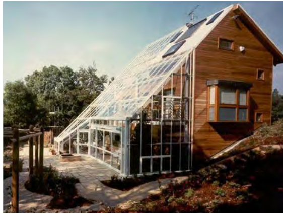
Above: BRE Integer House, Garston, Watford
