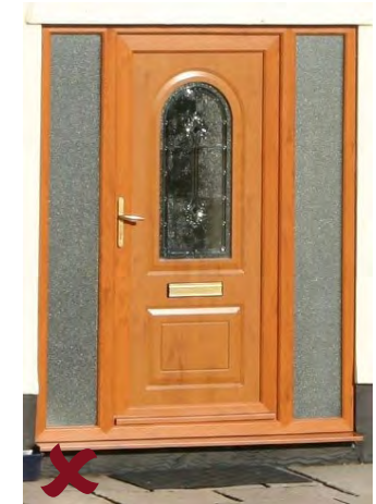
Above: poor example of doors - use of uPVC and resultant inappropriate style and details Below: good examples of doors - simple design, colour and choice of ironmongery
