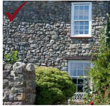
Above: traditional stonework with appropriate mortar colour and pointing detail
