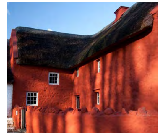
Below: Kennextone Farmhouse was originally covered with a limewash coloured with ox-blood
