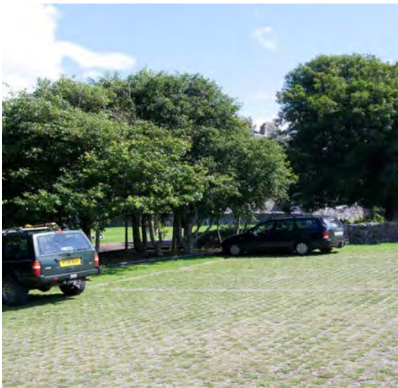
Above: understated reinforced grass provides visually soft parking area at Oxwich Castle
